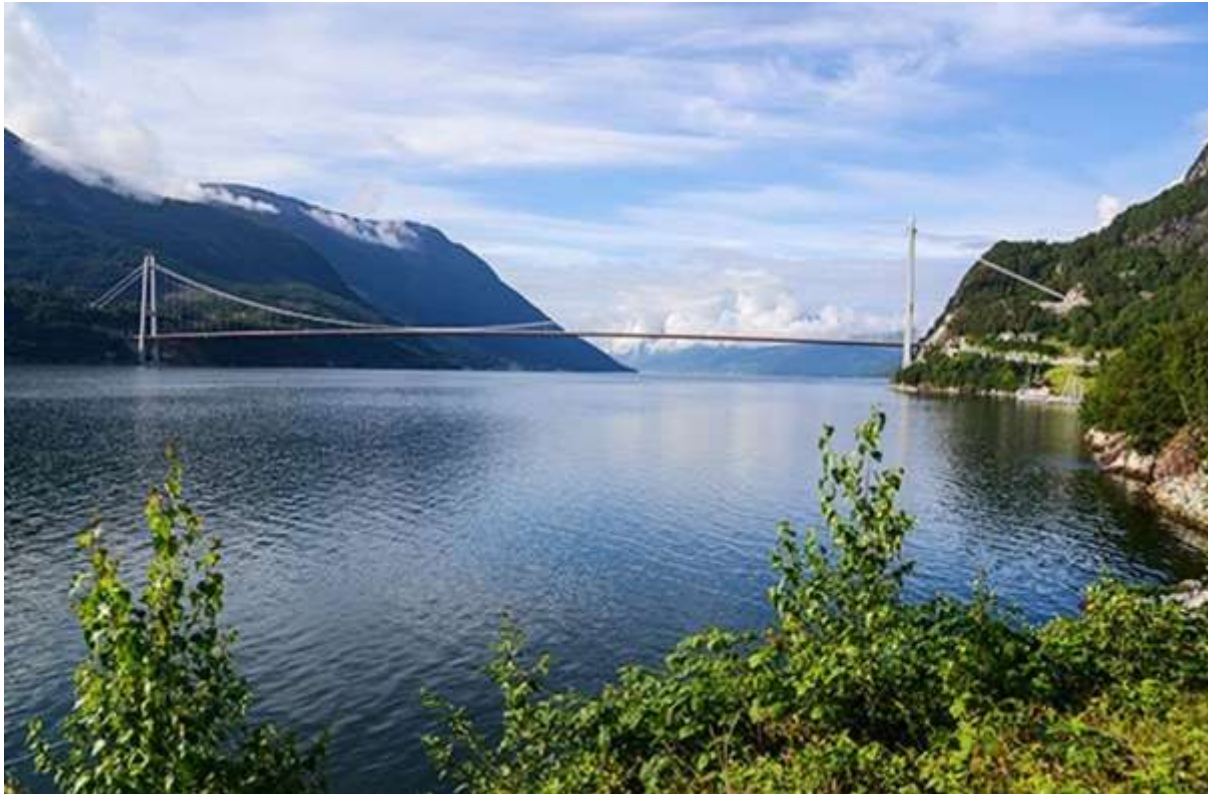
Hardanger bridge; 1380 m
